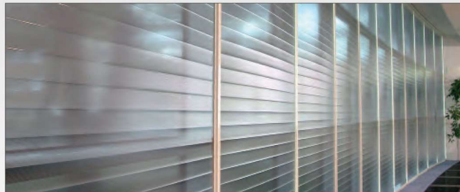
MULTIWAVE® pleating for high surface stability
